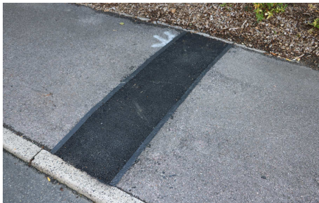
Patch Repairs
