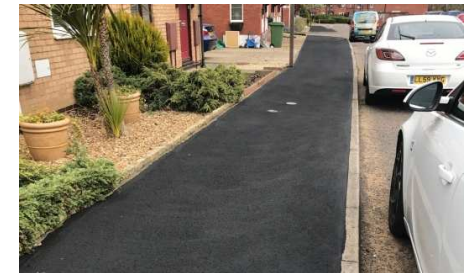
Slurry Overlay
